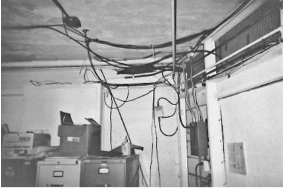
Grand Jury Photograph #7 - City Hall Basement (4/1/10)
