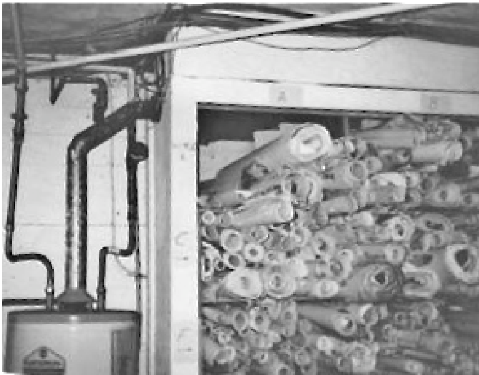
Grand Jury Photograph #8 - City Hall Basement (4/1/10)
