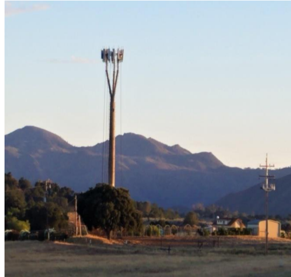
Tuesday, August 6 th , 2019 Tower Construction
