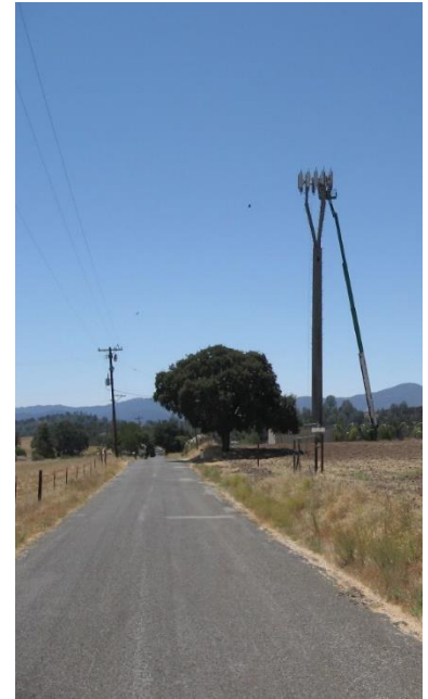
HESPERIA ROAD -- CELL TOWER CONSTRUCTION
