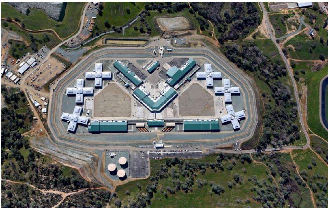
Overhead View of Infill Facility MCSP
