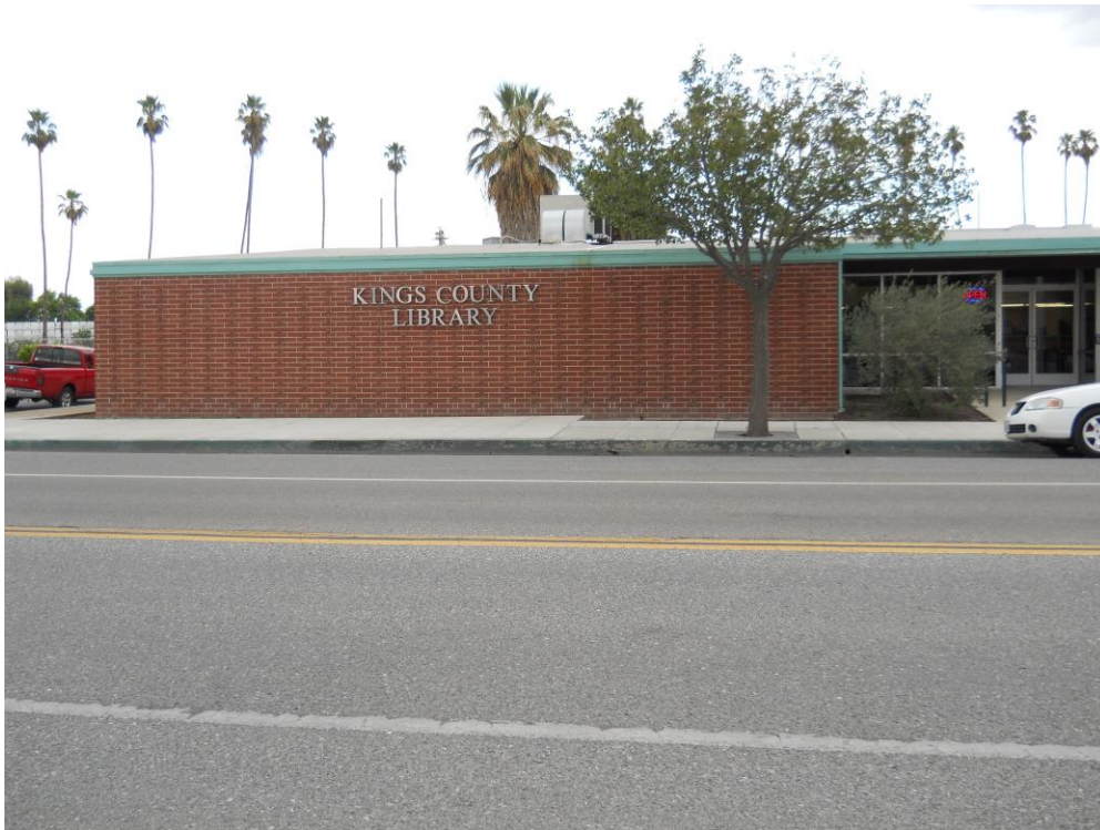
Corcoran Branch Library
