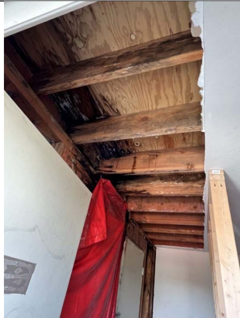
View inside abandoned training tower
