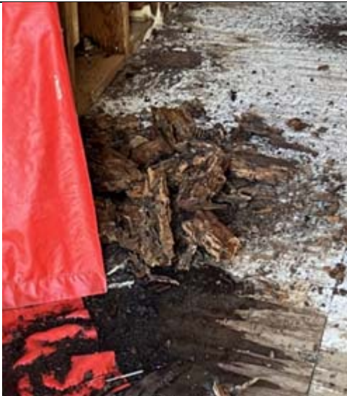
View inside abandoned training tower
