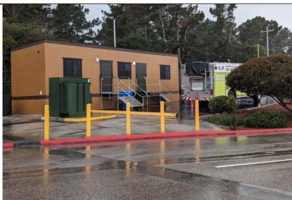
Modular trailer "fire station" at airport
