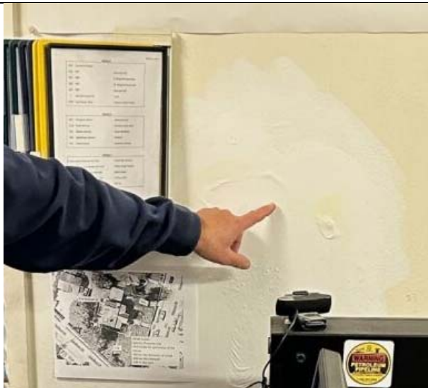
Bubbling paint after two weeks
