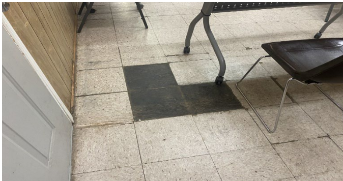
CEO mental health facility (photo provided by CEO staff)
