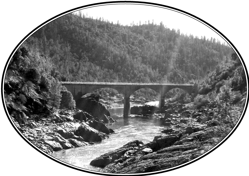
Mountain Quarry Bridge
