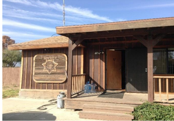
Figure 3 New Cuyama Sheriff's Substation
