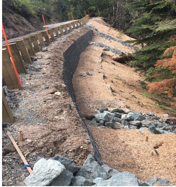
Shake Ridge Road Repair, March 2018
