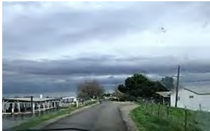
GJ photos: Pictures of levee crowns
