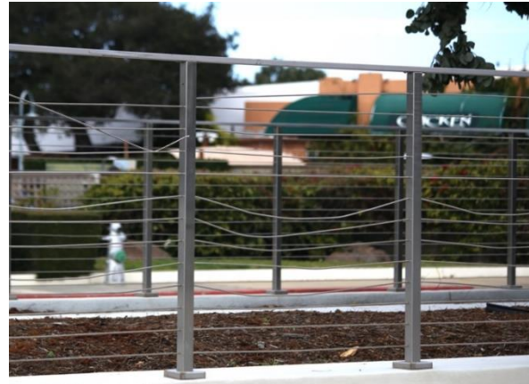
NFBPIP Railing: February 18, 2021
