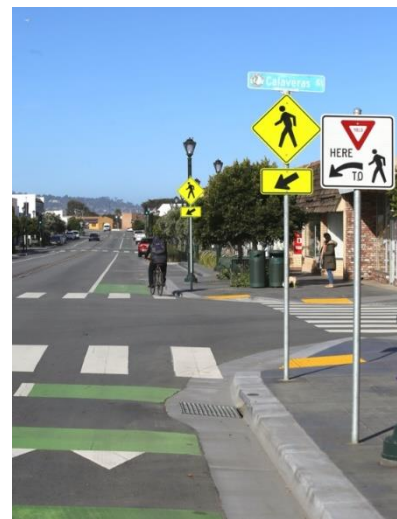
Seaside Project March 7, 2021
