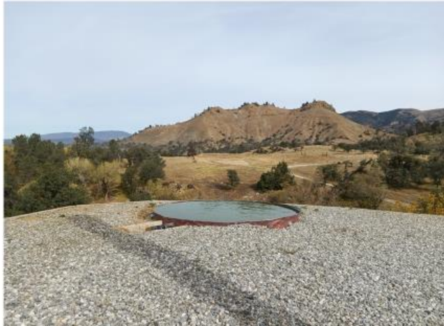
Photo provided by the Grand Jury (Station 11 Dip tank)
