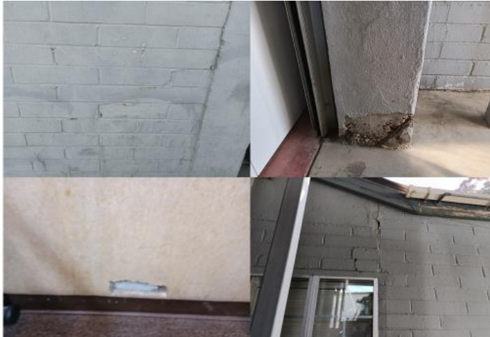
Photo provided by the Grand Jury (Station 45 building structure)
