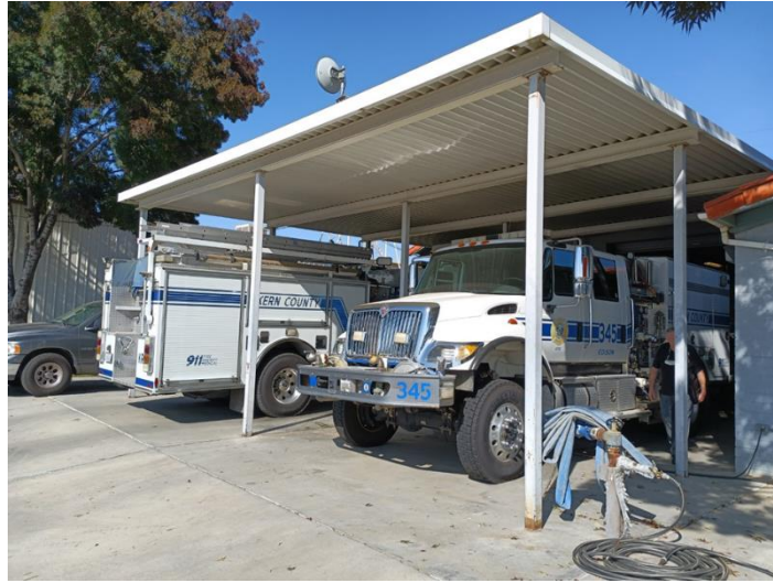
Photo provided by the Grand Jury (Station 45 garage extension)
