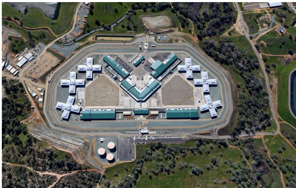
Overhead View of Infill Facility MCSP
