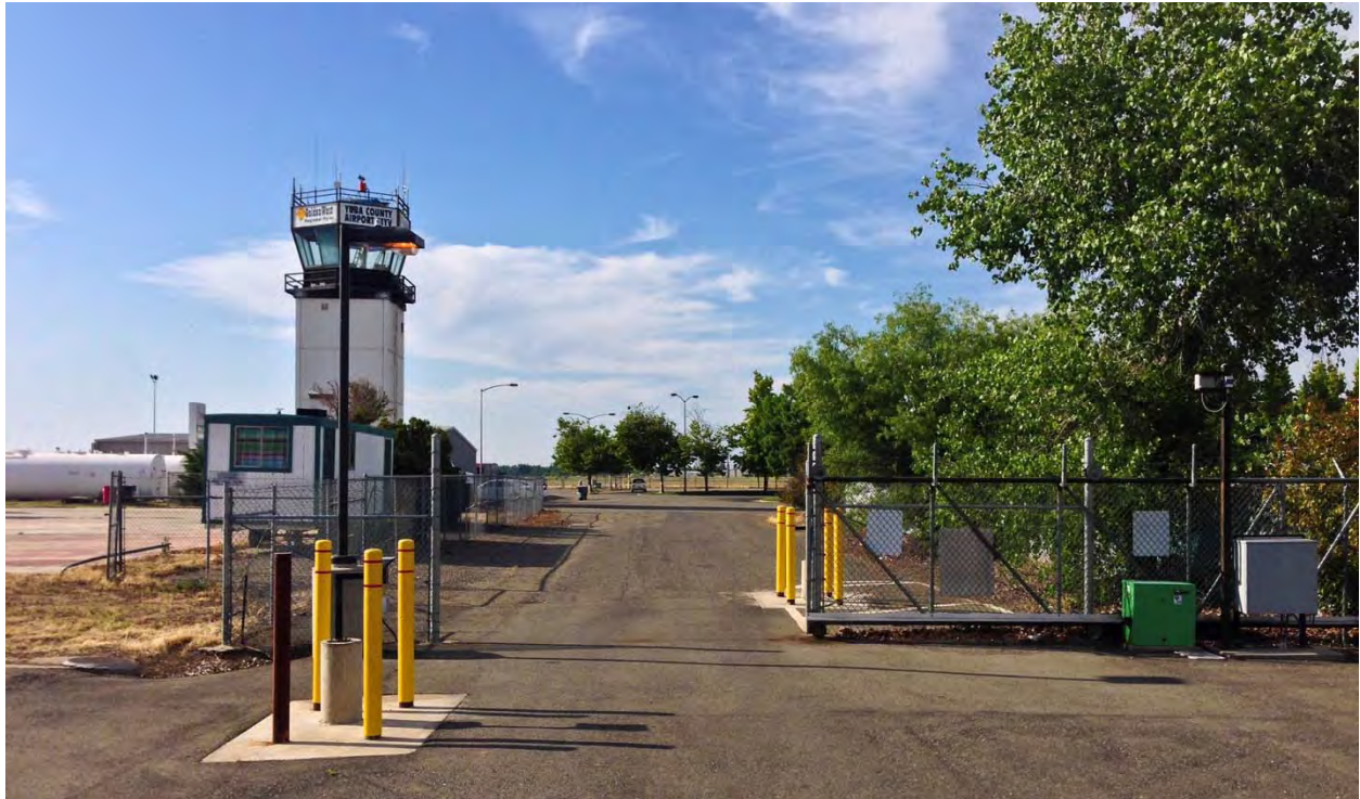
Figure 3. This is the main gate used for access to flight line and hangars. This gate was found open on the day the Grand Jury visited the airport.
