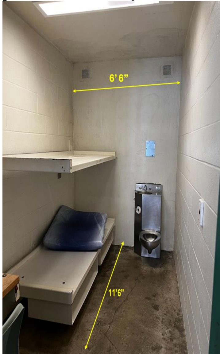
Figure 4: Interior View of County Jail Double Bunk Cell
