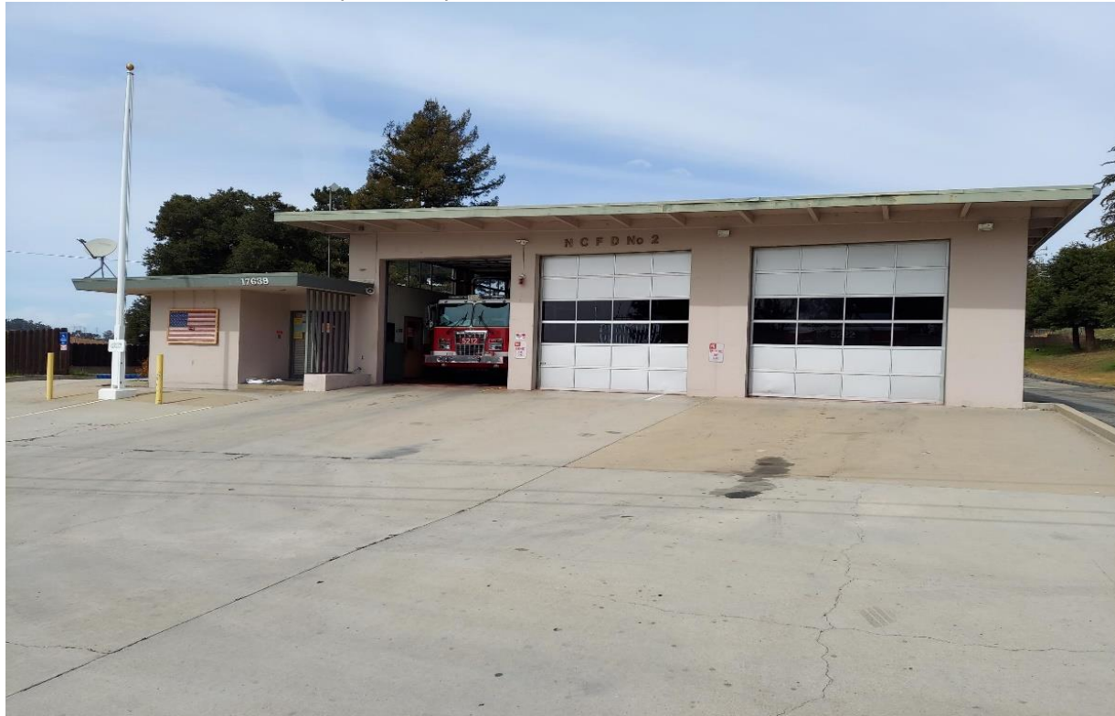
PRUNEDALE FIRE STATION (NCFPCD)
