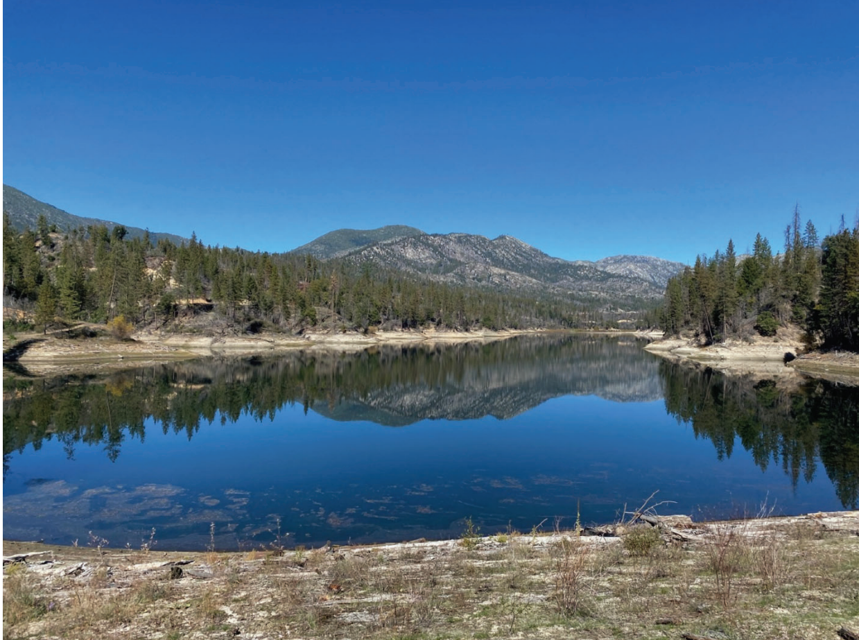
Rainbow Lake with restricted water level of 36 feet below spillway, October 2023. Photo taken from Misselbeck Dam.
