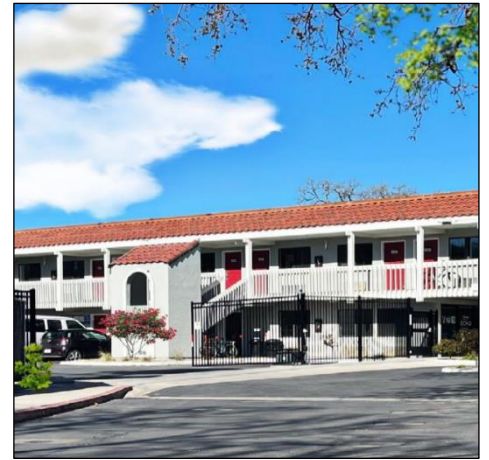
Converted Motel 6, Paso Robles
