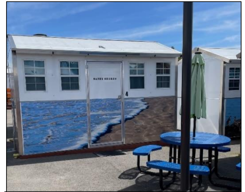
Cabins for Change, Grover Beach Location 1
