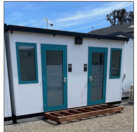
Cabins for Change, Grover Beach Location 2
