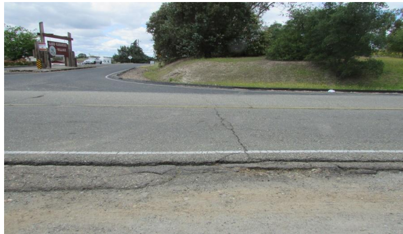
One of several small “dig-outs” on Curran Road which has been repeatedly replaced. Note pile of failed pavement to left of road.
