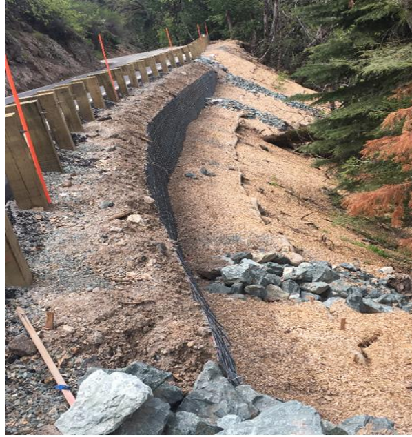
Shake Ridge Road Repair, March 2018
