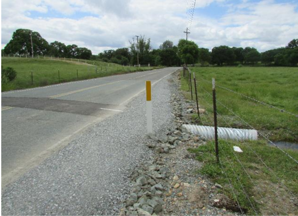
The eastern end of the .4 mile section with 16-18 transitions of section-replaced pavement. The culvert in this view is the recently replaced 18” one mentioned above.
