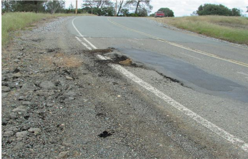
One of several small “dig-outs” on Curran Road which has been repeatedly replaced. Note pile of failed pavement to left of road.
