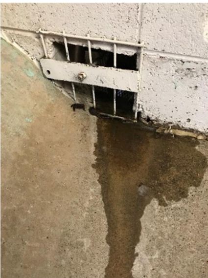
Fig. 1 - Floor drain in dog kennel area
