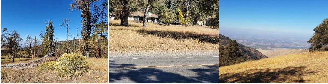
(Photos by the Grand Jury showing parcels within District needing hazard reduction, October 21, 2019)
