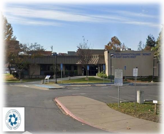
Peralta Community College District Office
