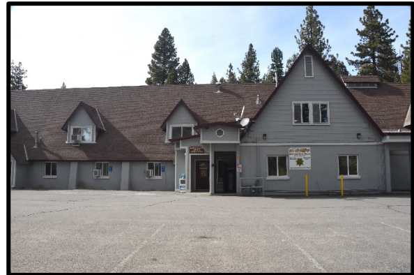
Tahoe Substation Photo by Jim Ferguson
