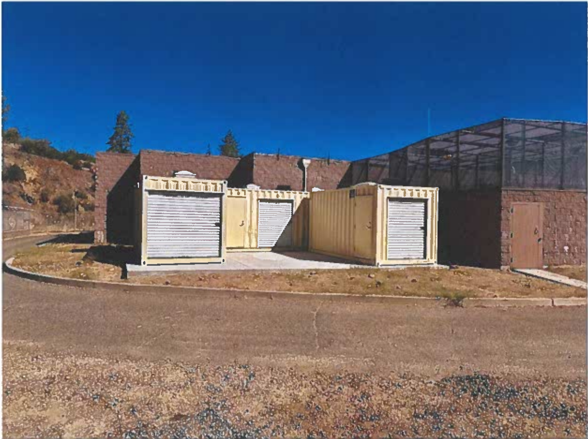
Image 1: Storage Containers at Mariposa Adult Detention Facility installed for the purpose of extra storage in order to maximize office space for jail staff inside the main building.
